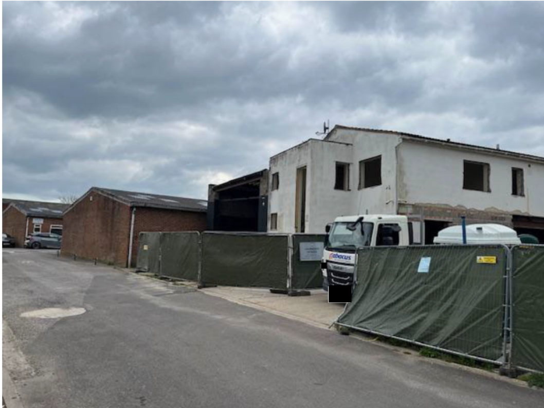
5. Side of Tesco site, opposite photograph. Photograph shows small business premises at the rear
